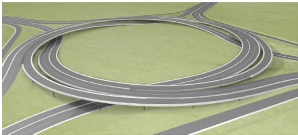
Fig. 5. Two-level Pinavia interchange of four roads
