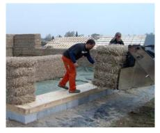
Fig. 7. Construction using big bales, Denmark. Photo by Lars Keller
