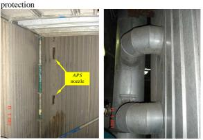
Fig. 3. APS nozzles in boiler OP-230 (K-6)
