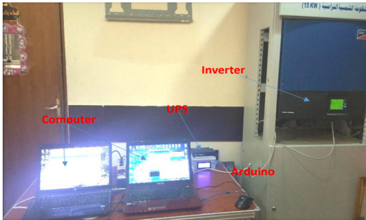
Fig. 5. Grid-tied solar inverter (SMA-SUNNY TRI POWER 15000 TL)
