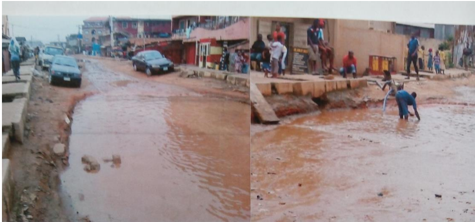
Fig. 1. Road/drainage upgrading works in Agege area of Lagos
